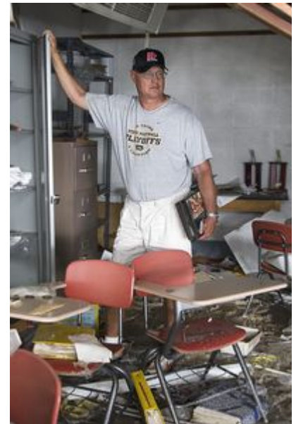
Football coach Ed Thomas surveys damage in the school.
